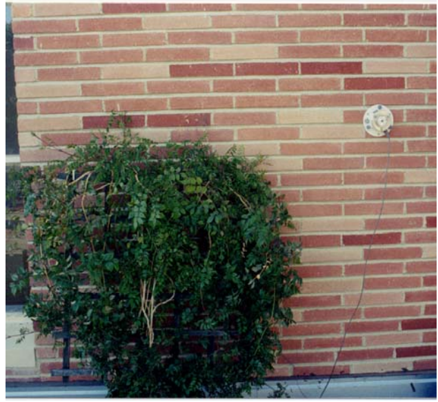
Fig. 2- Campsis vine on a South facing brick wall
