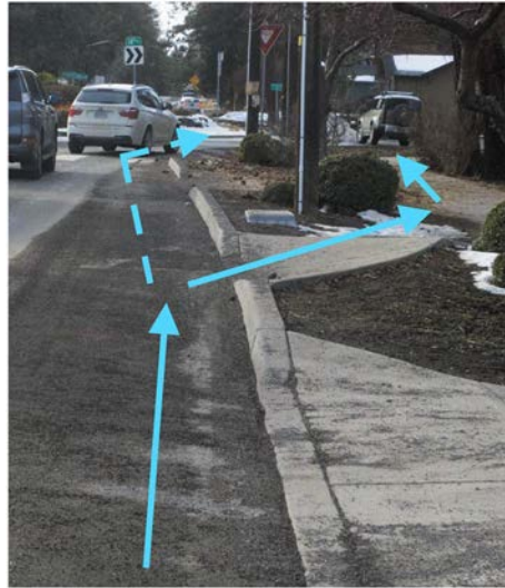
Bike lane curb cut to sidewalk.
