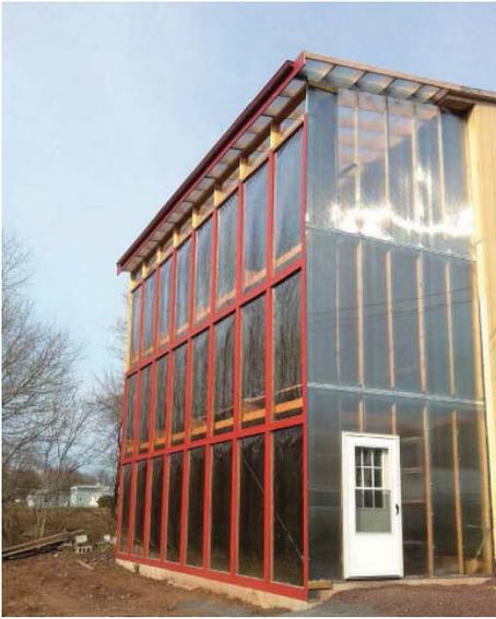
The Pine sun space shows off its clear polycarbonate east and south façades and its double-mesh inner layer.
