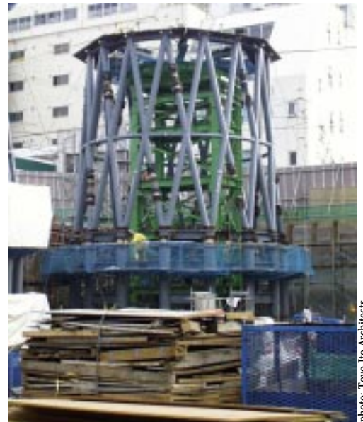
The latticed steel structure of Ito's Sendai Mediateque under construction.
