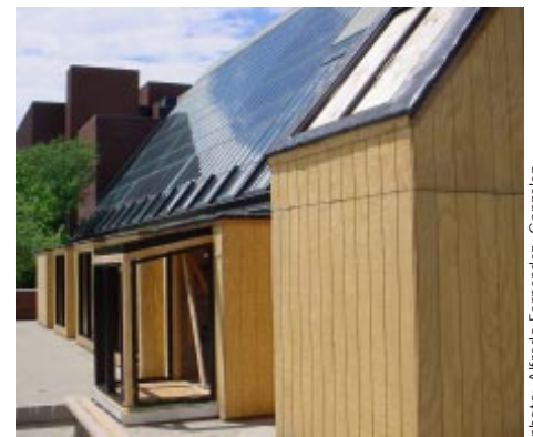
Six test cells (Control, DG, TW, WW, SS, and Skytherm North with the pitched roof) under construction on the architecture terrace. [Are they permanent or emergency faculty offices?—ed.]
