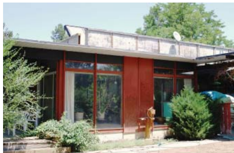
Löf's collectors (partly visible behind plywood screens) simply consisted of clear glass, airspace, black aluminum, and insulated backing
