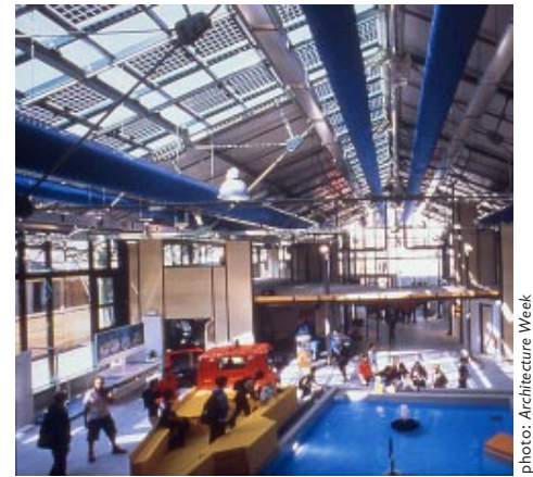
Is the Children's Museum in Rome an example of the best use of PVs? Its PV-integrated skylight helps avoid electric light use by day while providing electricity to the grid.
