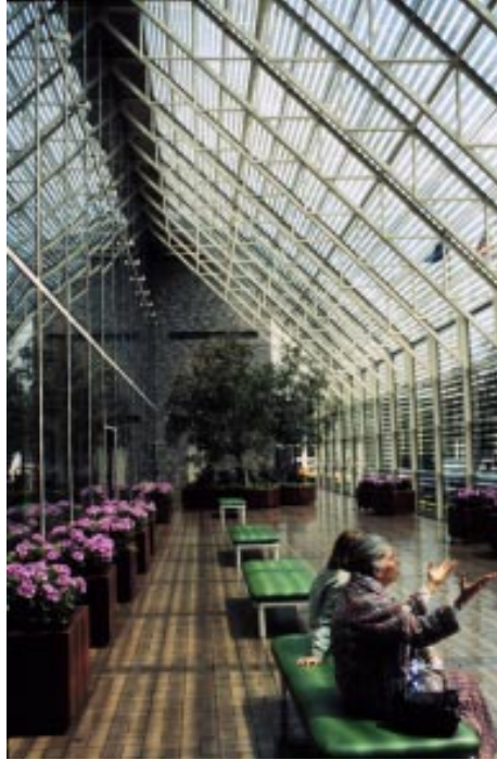
Columbus' Irwin Union Bank & Trust Company Arcade Addition (1973) by Kevin Roche features "striped" glass, a laminate of two layers of glass, one sprayed in stripes with a reflecting substance similar to that used to back mirrors.
